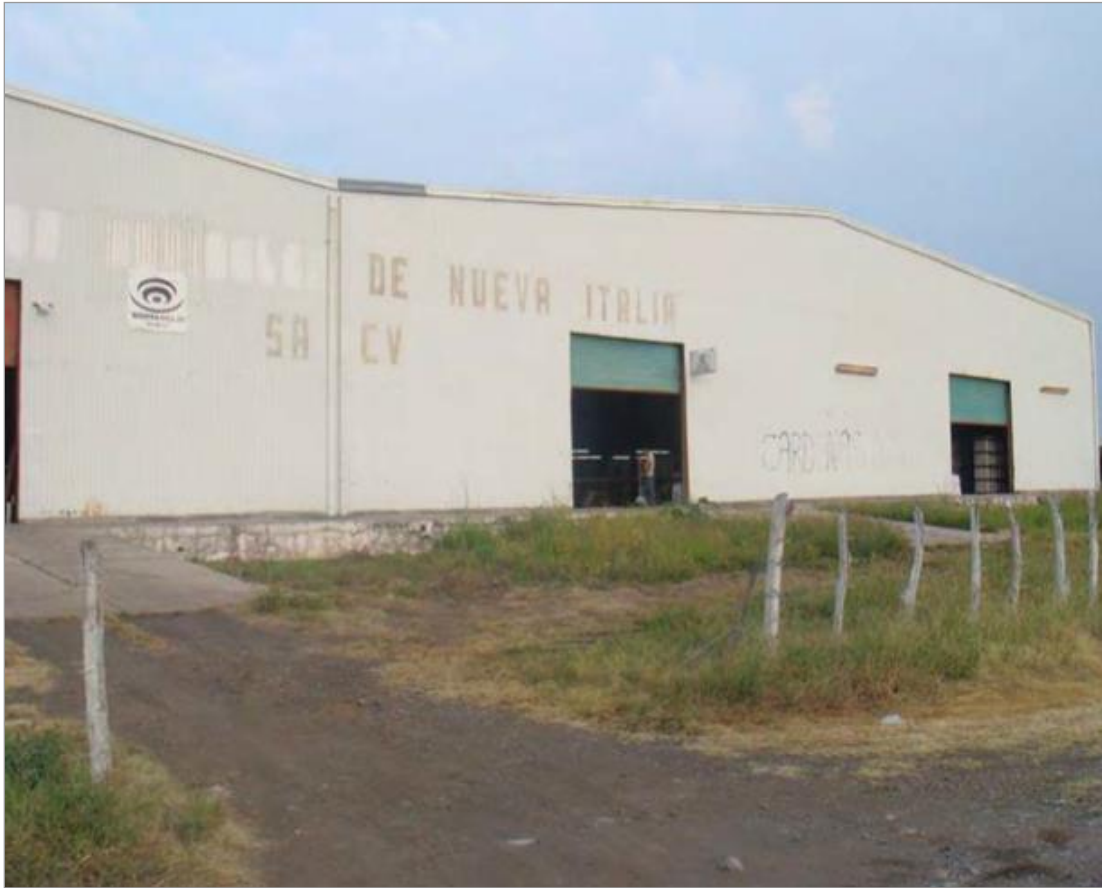
Figure 5.1 Lowell copper core storage and sampling facility
