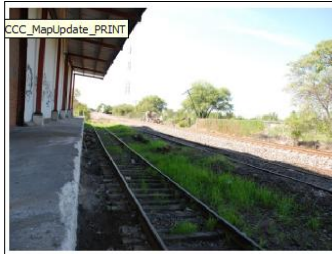
Figure 18.5 Active Rail Transport Close to Core Shack
