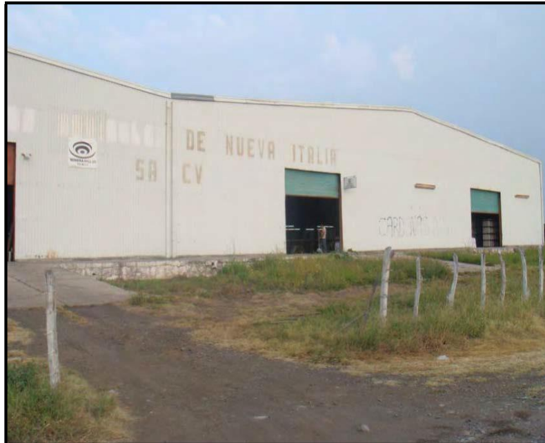
Figure 5.1 Catalyst Core Storage and Sampling Facility
